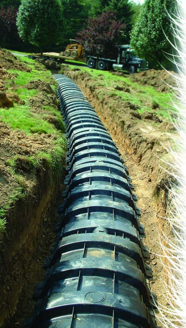
Alternating drainfields provide relief for a failing system. Here, a second drainfield is installed.
