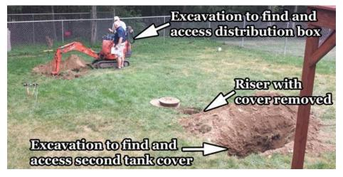
This is a picture of a septic system with only one riser. As you can see, the inspectors required an excavator to dig down to the septic tank and distribution box access covers. This
